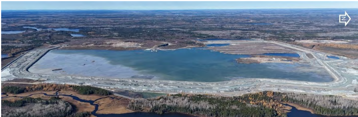
Figure 18-1: Tailings Management Facility (October 2025)
